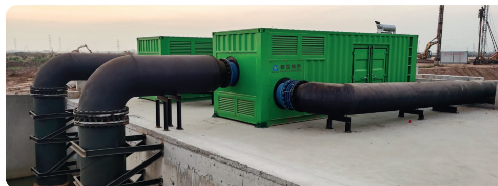
Container Pumping station drainage project site
